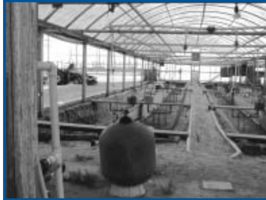
A greenhouse-enclosed raceway used in a nursery with limited discharge.
